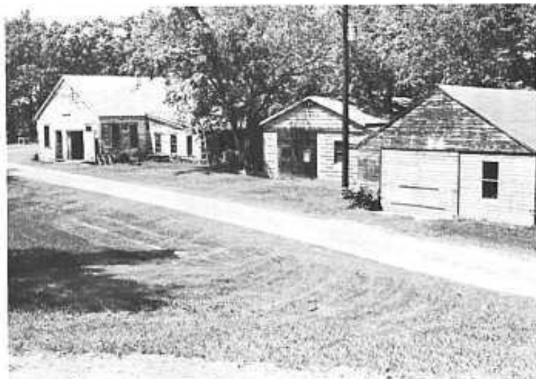
Above: Shade trees and weathered shop buildings
