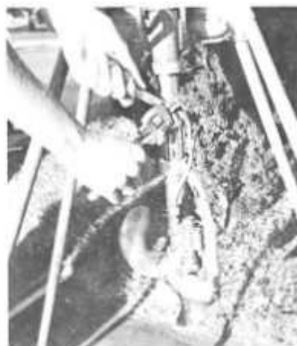
Figure 1: Loosening the 90 degree elbow.
