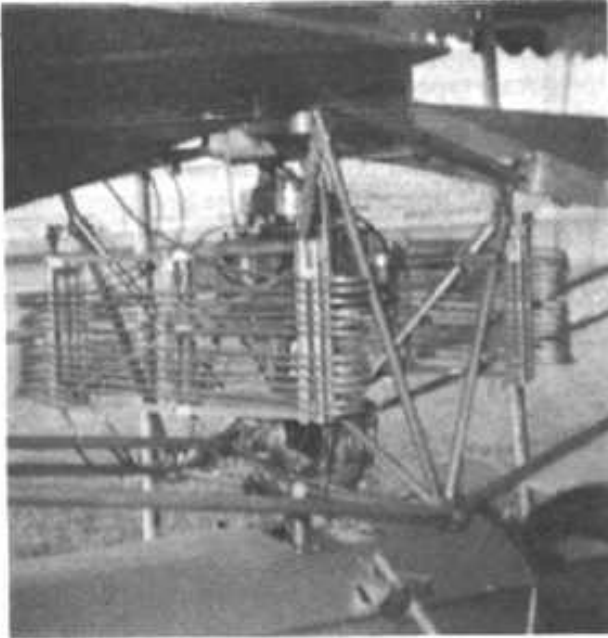
Near the top can be seen the gas tank with the word Halligan on it. Note "radiators" and pump to right of differential.
